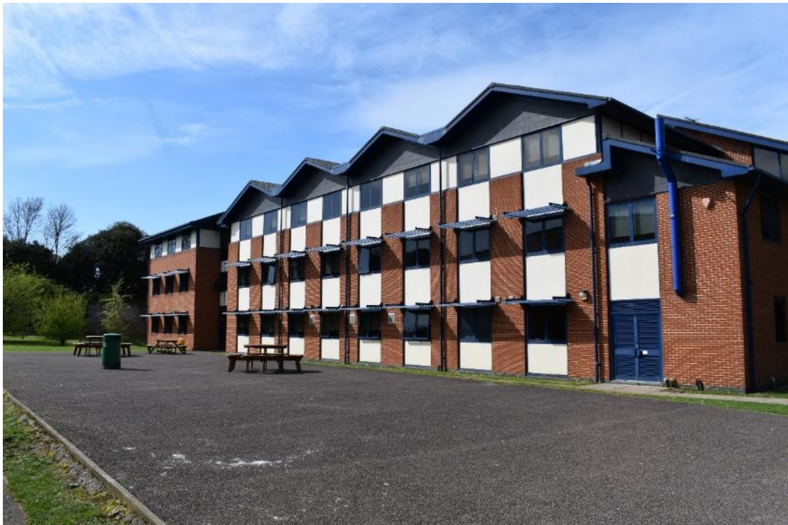
Plate 17: View of the rear of Block B (facing NW)
