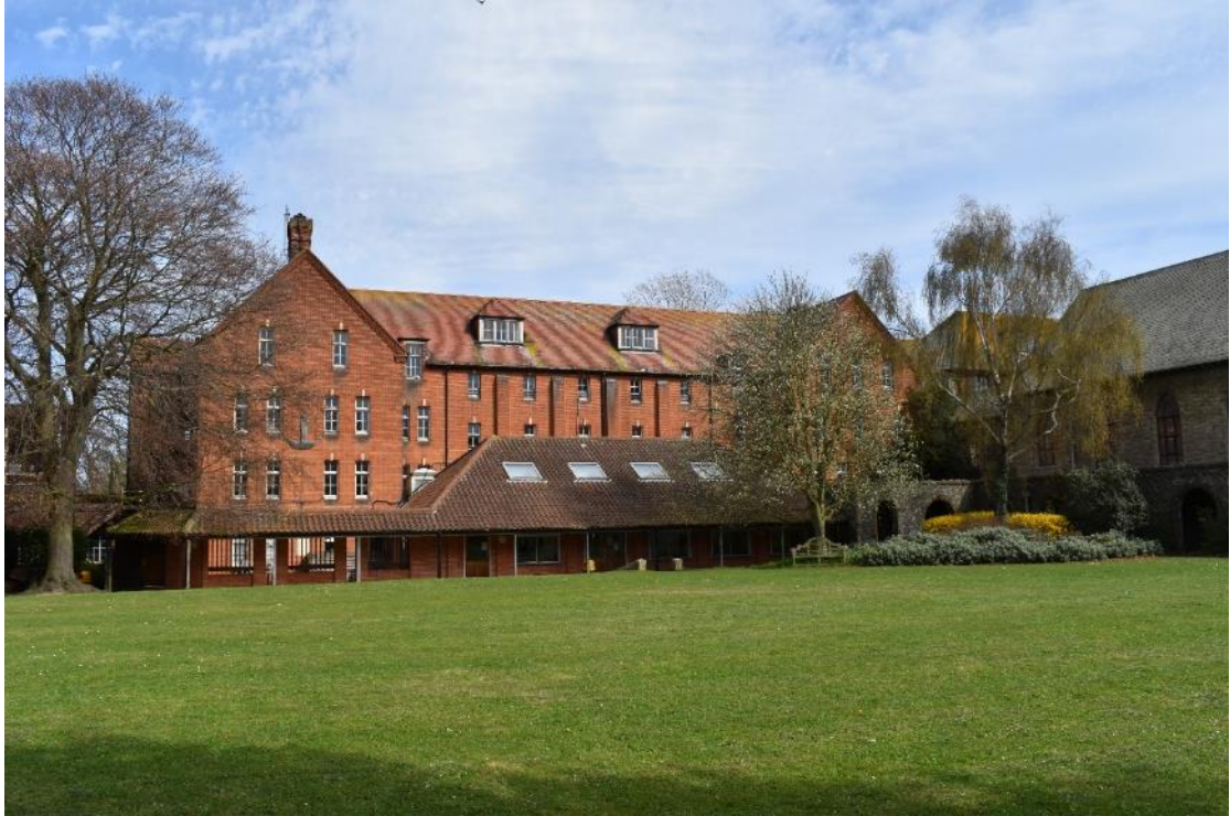
Plate 14: View of the front of Block C (facing E)
