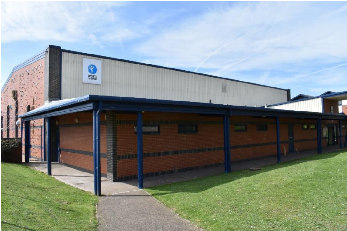
Plate 19: View of the sports hall (facing NW)
