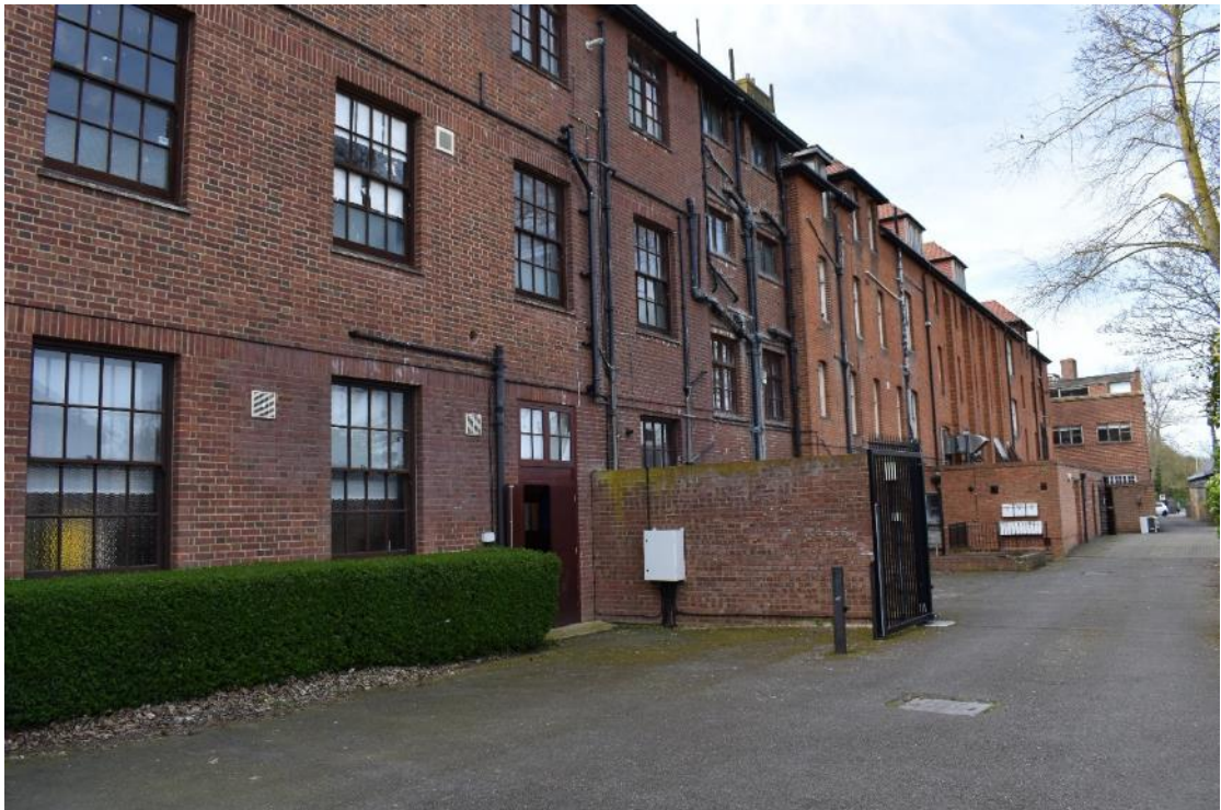
Plate 15: View of rear of Block C both the original 1907 section and the 1930s extension (facing NW)
