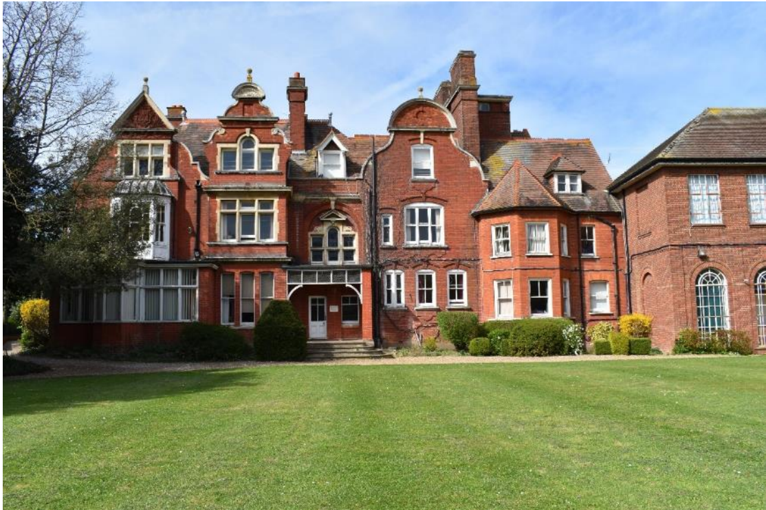
Plate 12: View of the rear of Hatton House (facing NNE)
